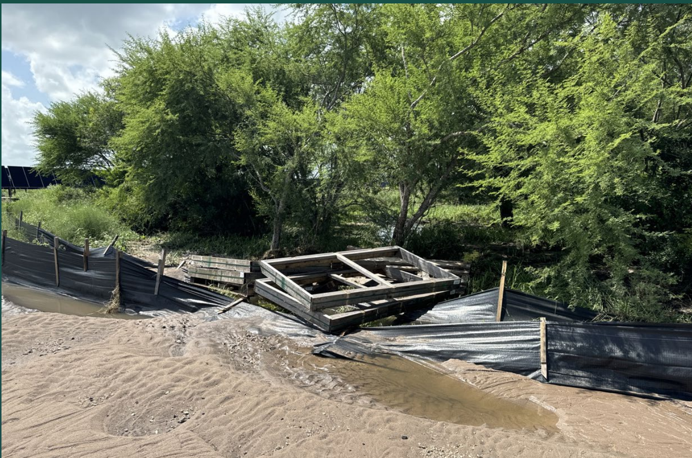
Silt fence surrounding a wetland on an active solar construction site in Texas. Construction monitors play a vital role in identifying BMP deficiencies and mitigating environmental impacts in real time, helping to protect sensitive ecosystems like wetlands.
